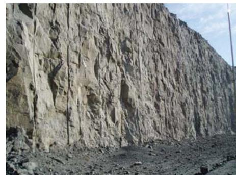
Figure 3—Single-pass 28 m pre-split on basalt
