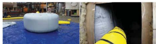
Figure 10—Duct balloons used for isolation
