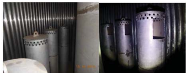
Figure 7—Bed 4 bypass caps before and after modification
