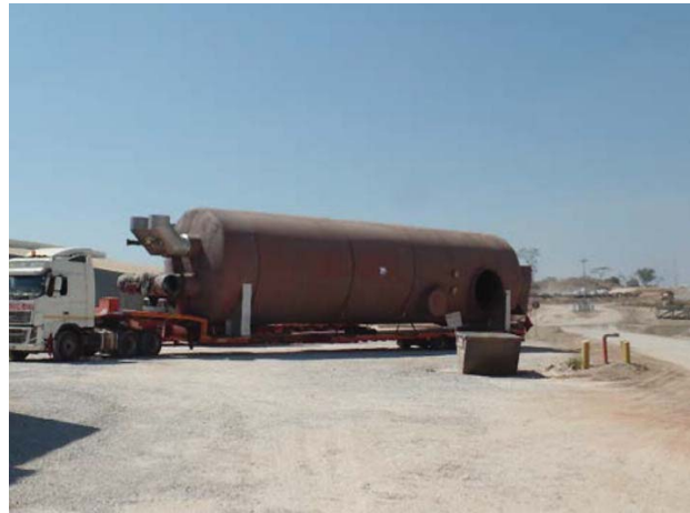
Figure 4—Sulphur furnace shell delivered to site
