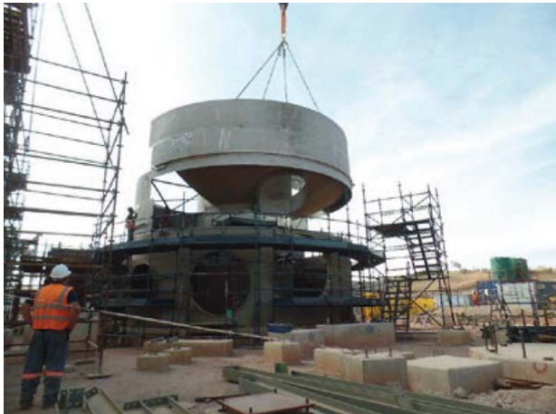
Figure 8—Converter modules assembly on site
