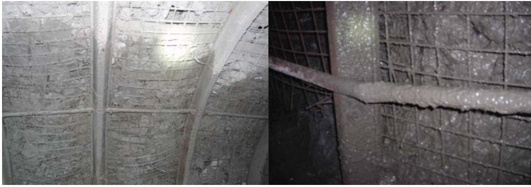
Figure 2—Application of ash, cement, and water mixture to prevent spontaneous combustion (Onur et al. , 2012)
