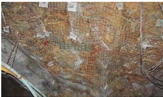
Figure 22—Hammock-shaped straps installed underground
