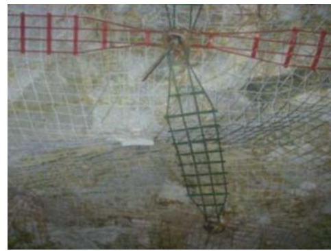
Figure 18—Underground installation of a hammock-shaped Osro strap
