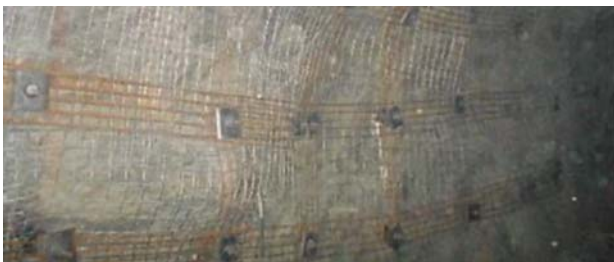
Figure 2—Eccentric loading of Osro straps underground
