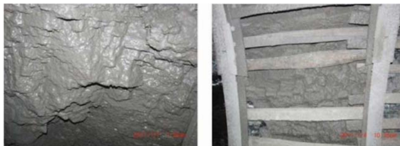
Figure 7—Application of cement, fly ash, and water mixture between two supports
