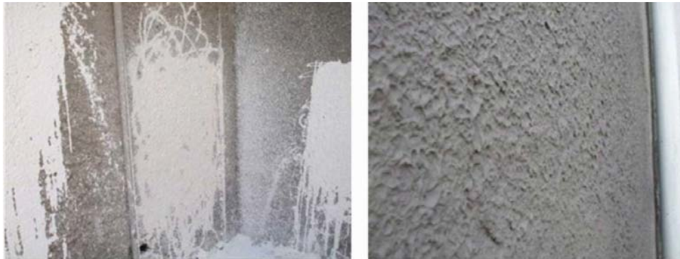
Figure 4—Mixtures sprayed on wall
