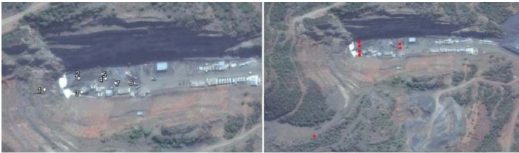
Figure 6—UAV surveyed points
