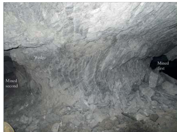
Figure 8—Fracture pattern along the width of failed crush pillar 19
