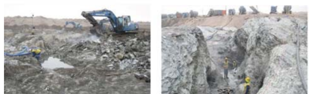
Figure 6—Photos of bedrock operations, showing bulking on the left and some very deep bedrock gullies on the right
