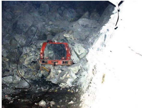
Figure 8—A TORO LH514 LHD in an open stope, damaged by a fall of ground (le Roux, 2015)
