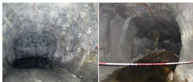
Figure 11—(a) HPS development with bolts and mesh (b) HPS development with fibrecrete
