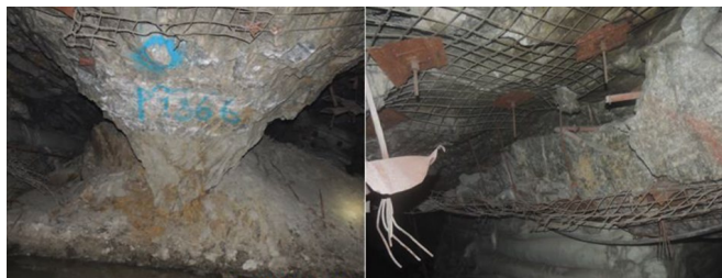
Figure 8—(a) Deteriorated crush pillar in LPS (b) Opening of bedding planes in LPS
