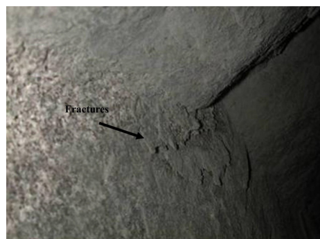
Figure 19—Fracturing in the sidewall looking northeast up the raise
