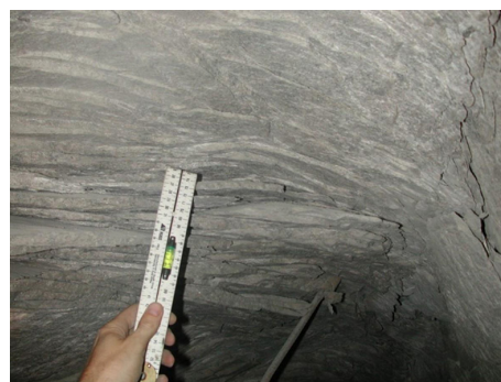
Figure 18—Extensive fracturing in the anorthosite, in the hangingwall of the raise
