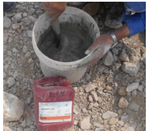
Figure 4—Stemming plug 3 (mortar preparation)
