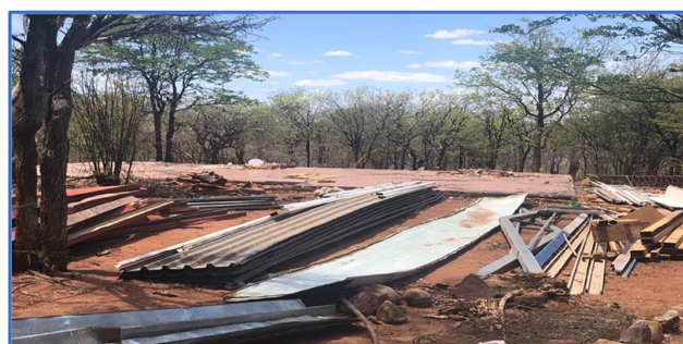
Figure 8—Demolished prefabricated house at Tshikondeni mine village
