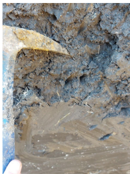
Figure 2—Typical test pit profile of the reworked residual norite with the presence of slickensides
