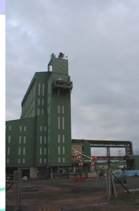
B11 to be installed outside of furnace building to allow for safe escape of gas
