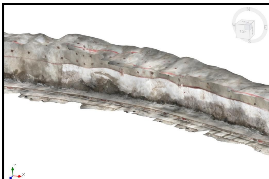
Figure 3. An underground i-Phone scan 3D model of a haulage with tracks
