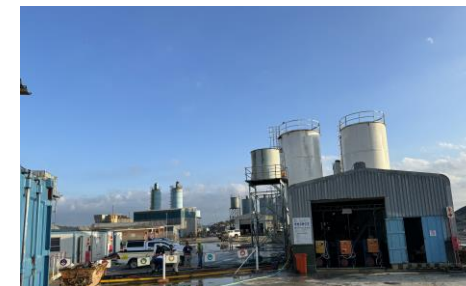
3 Pump Grout Plant set up for our client's production requirements
