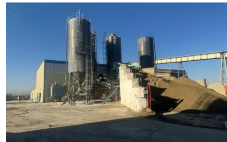
Upgraded to 8 Pump Grout Plant
