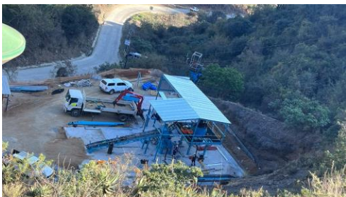
3 Pump Grout Plant being set up for our client in the mountains
