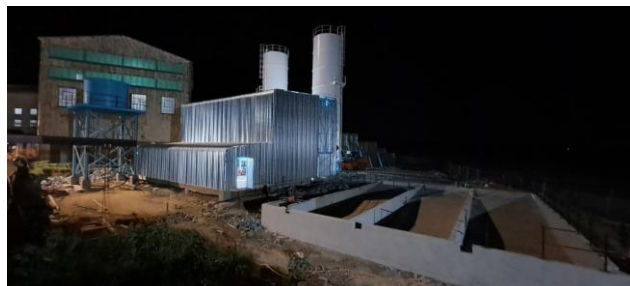
8 Pump Grout Plant delivering 12000 Cubes per month
