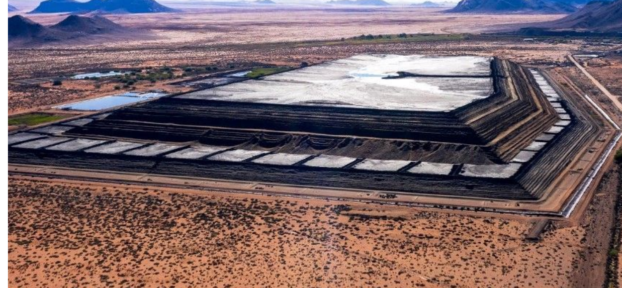
Gamsberg Tailings Storage Facility (International Mining, 2021)
