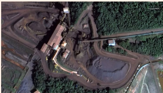
The dam at Vale's Corrego do Feijão mine near Brumadinho pictured in a satellite image before its collapse © Reuters
