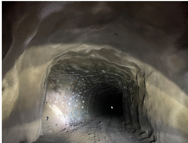
Figure 2: Supported ground with shotcrete, mesh, straps and bolts in Western Australia.
