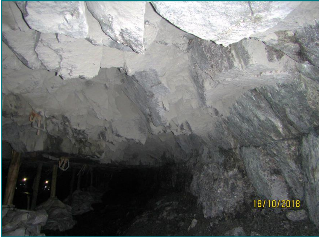
Before blast-on mesh
